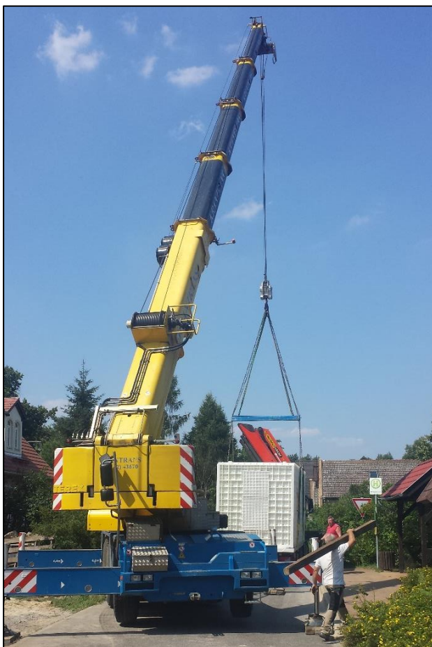
Installation of the system on site in Vetschau
