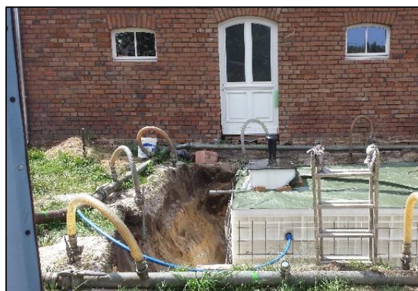
Installation of the polyethylene module below ground
